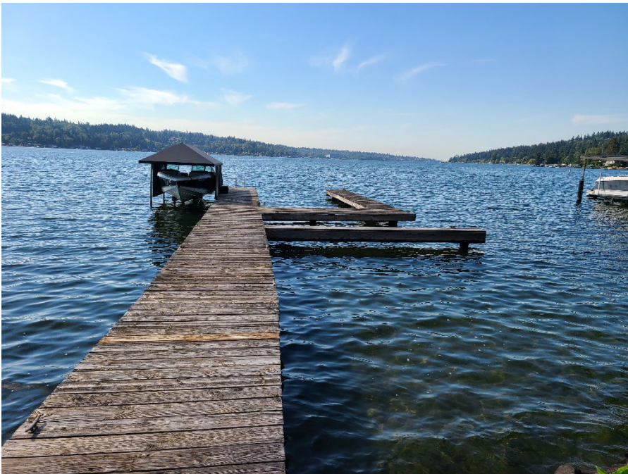
Photo 2. View looking southeast of existing dock proposed to be replaced. Note existing wood decking.
